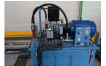
Hydraulic power unit
